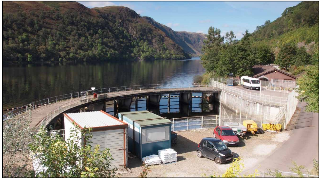
Cruachan tailrace at Loch Awe and the visitor centre building: the site hosts invertebrates and a breeding bird assemblage
